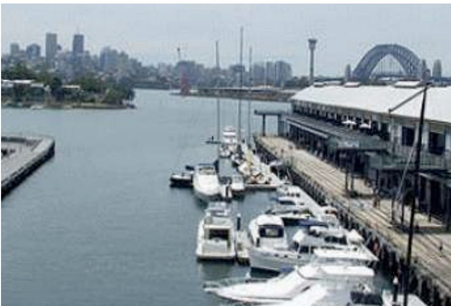
Jones Bay Wharf, Pyrmont
